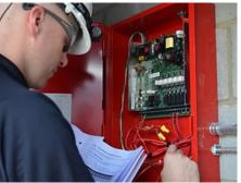
• **Every five years:** Zoned fire alarm system smoke detectors shall be sensitivity tested. Addressable smoke detectors can be verified through fire panel programming.
